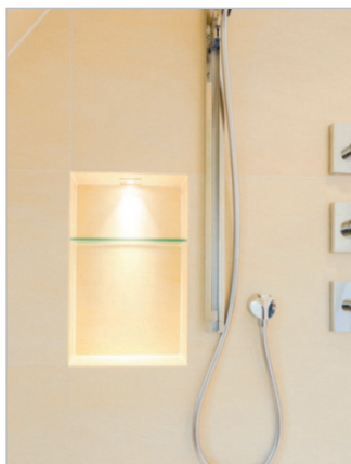
■ The installation of different lighting systems is easily doable, if the duration of temperature is not above 75 ° C.
