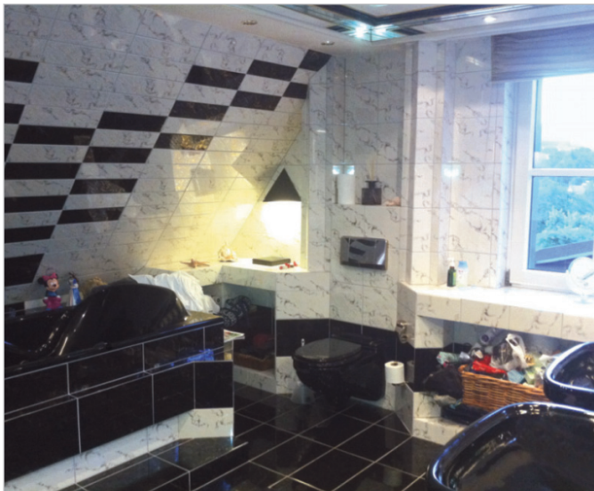
■ OLD – roof slopes, dark floor tiles and black bathroom ceramics made the room look dark and heavy.
