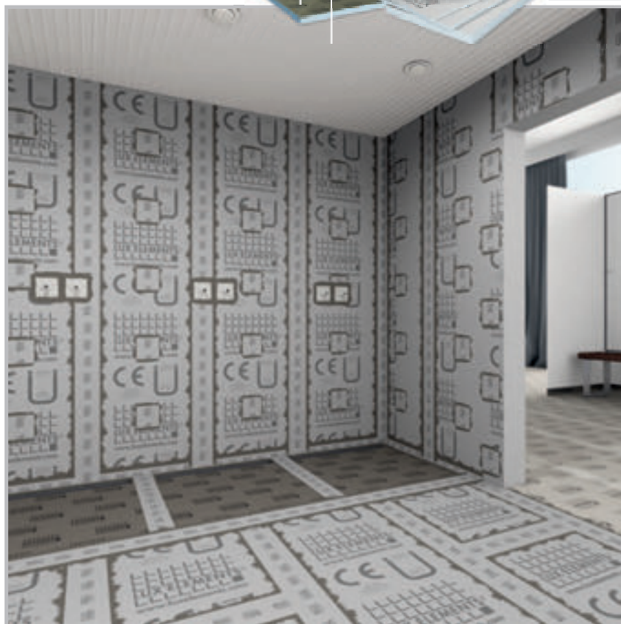
Shower area with sealing in a panel-shaped form
