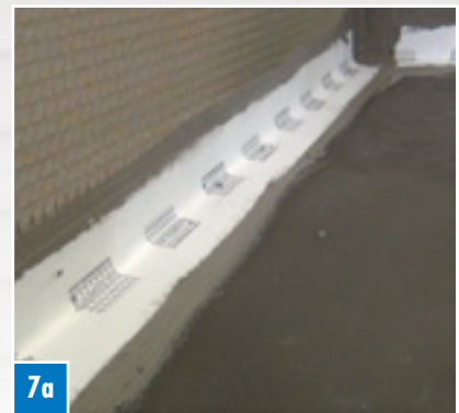
7a The surface is now ready for tiling or plastering.
