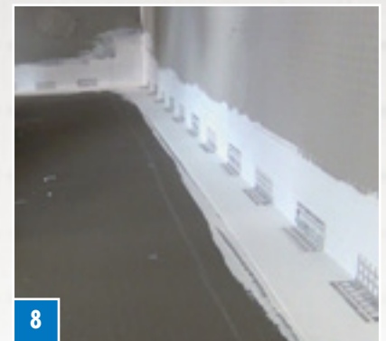
8 The surface is now ready for tiling or plastering.
