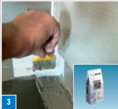
3 In the second step the joint is levelled out using DRY-ASK sealing filler.
