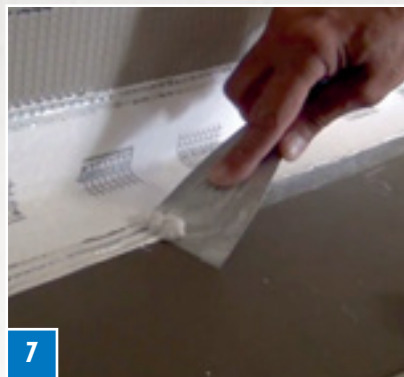
7 Remove excess adhesive.
