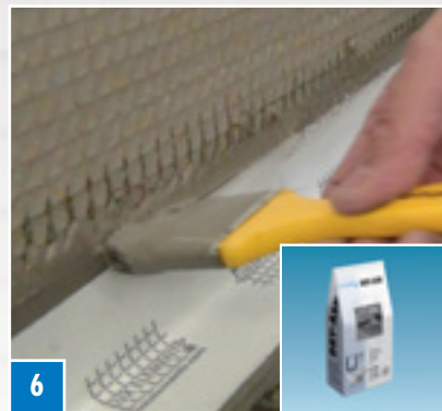
6 Level out the adjacent surfaces and joints using DRY-ASK sealing filler.
