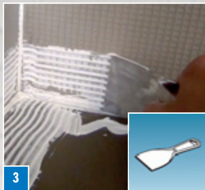
3 ... and spread it using a notched trowel.
