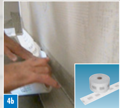
4b ... with DRY-ASK sealing filler and DRY-DB sealing tape.
